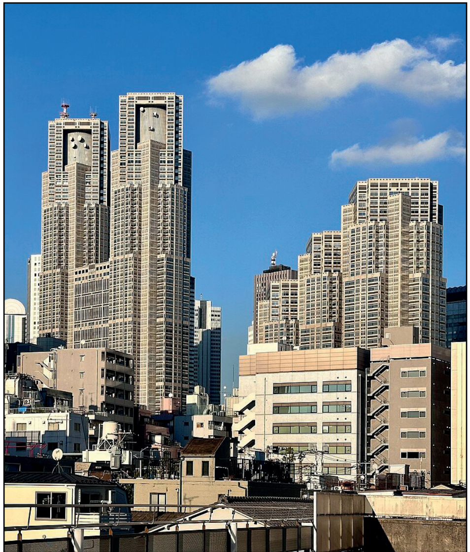
Tokyo Metropolitan Government Building (Source: Wikipedia).
